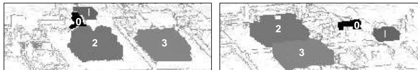
Fig. 5. These two images represent a power-plant complex seen from two different viewpoints. A fuzzy scene matching approach based on force histogram computation makes it possible to coherently label the buildings, and to retrieve the declination angles and the rotational difference.
